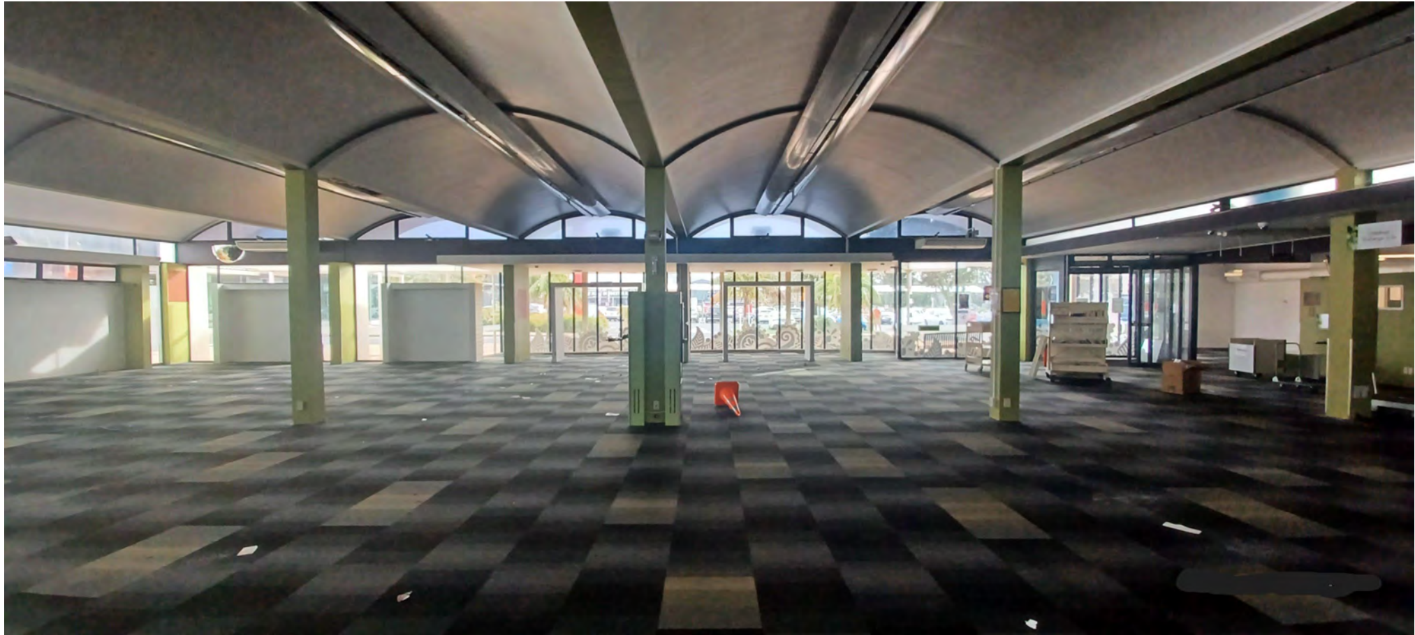
Orewa Library – All cleared out ready for refurbishment
