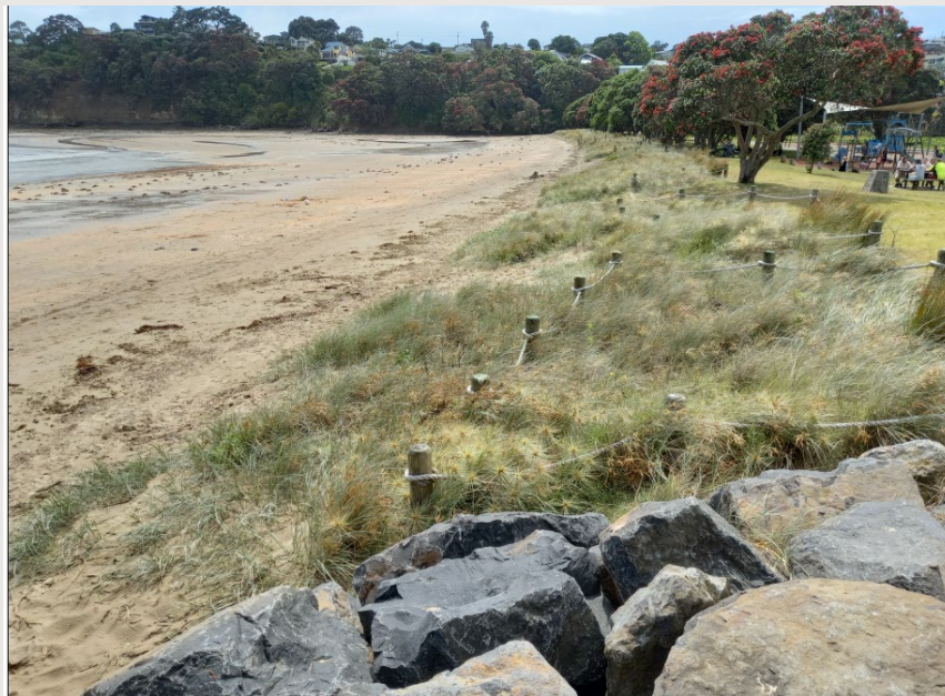
Above: Example of a formed and planted sand dune as a natural defense alternative in Stanmore Bay.
