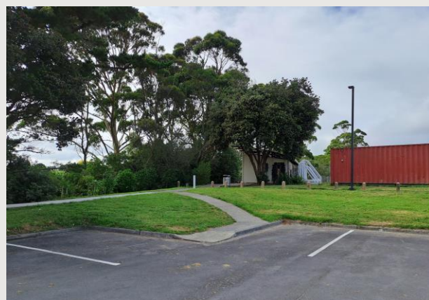
Existing toilet amenity adjacent to the car park
