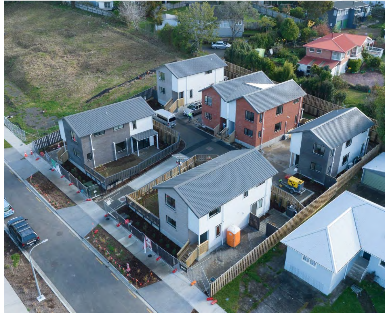
Completed Kaka St Social housing (6 new homes)
