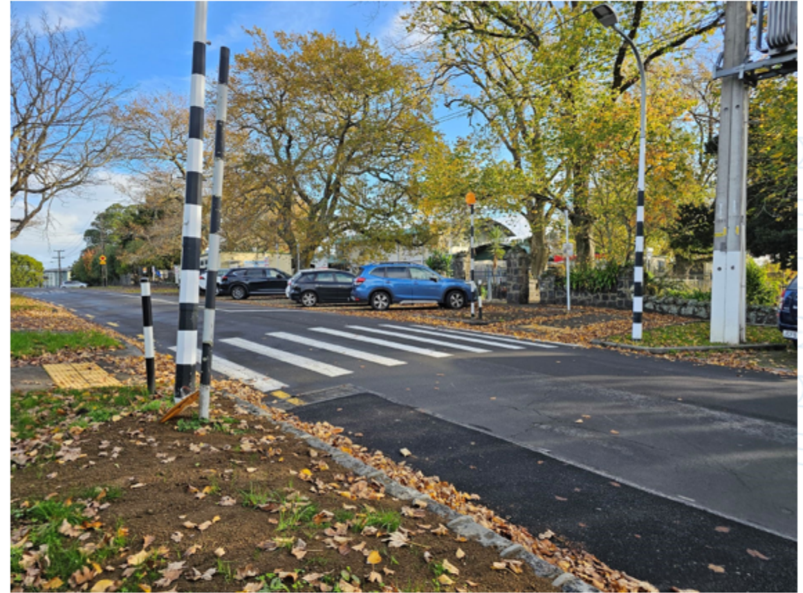
Site location – existing crossing
