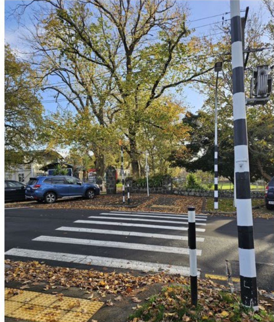
Site location – existing crossing
