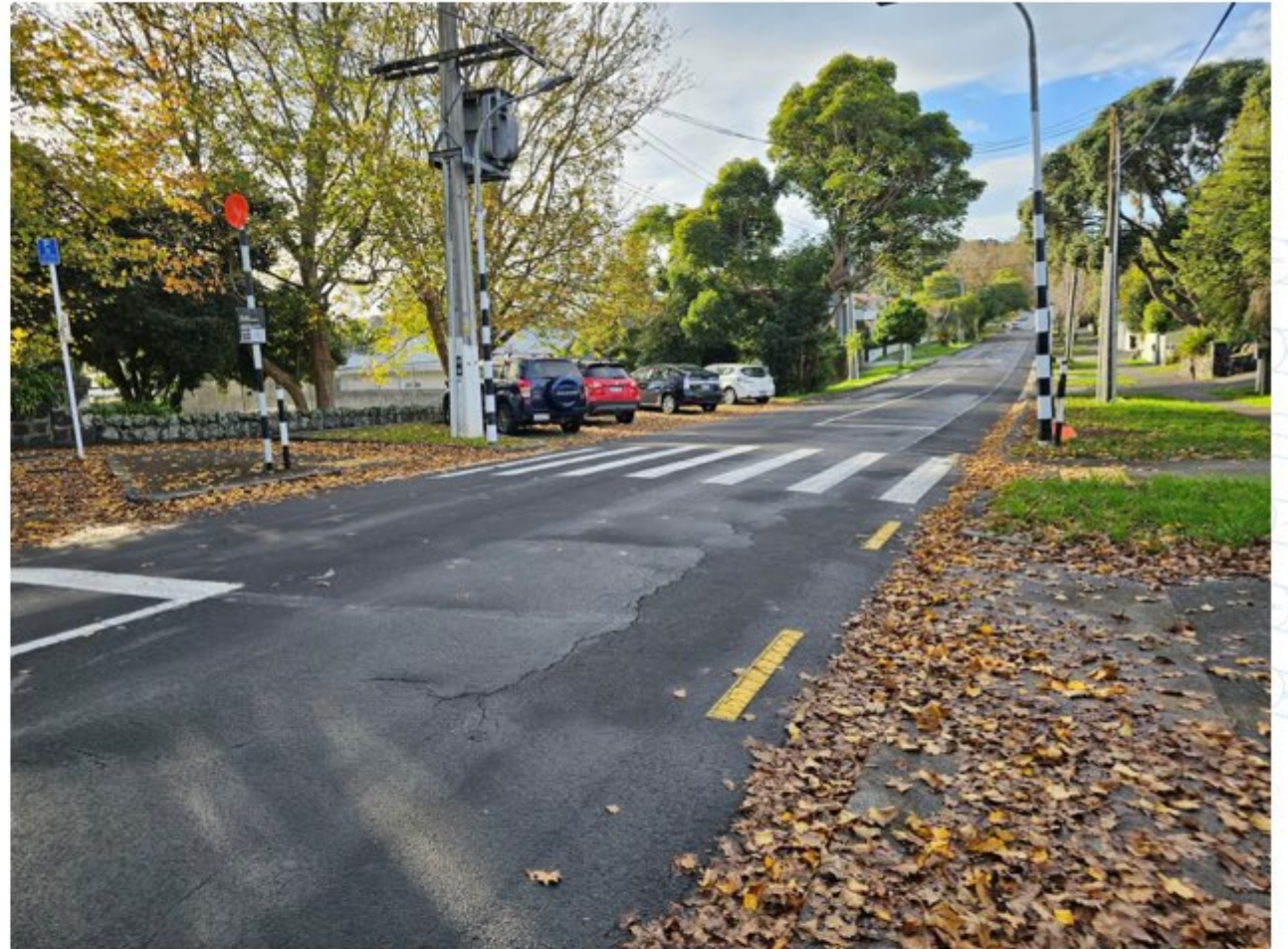
Site location – existing crossing
