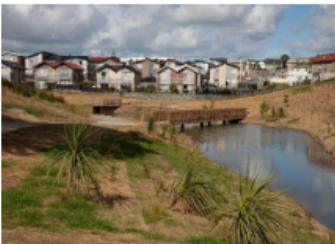
Freeland Reserve upgrades
