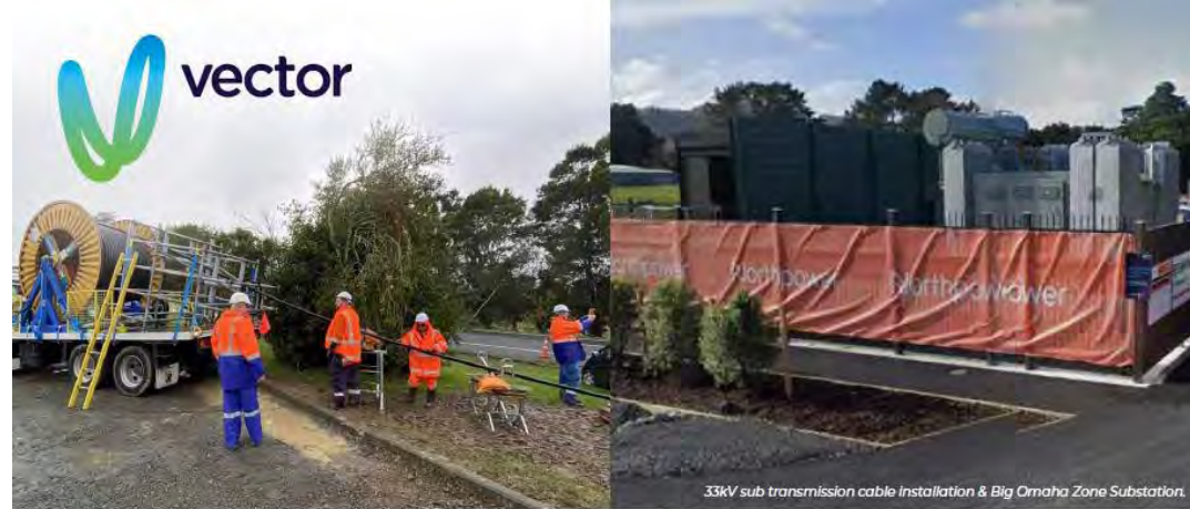
33kV sub transmission cable installation & Big Omaha Zone Substation.
