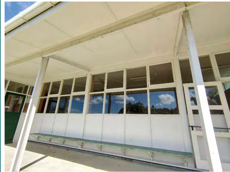
14. Exposed steel portal frame (side span) of the east corridor
