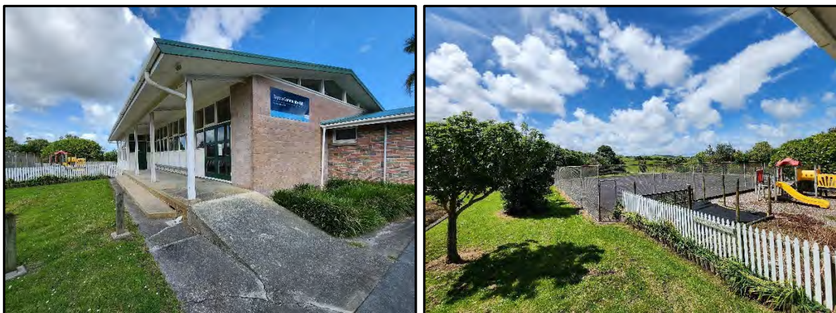
Photos 1 & 2 Existing hall building and outdoor court facility
