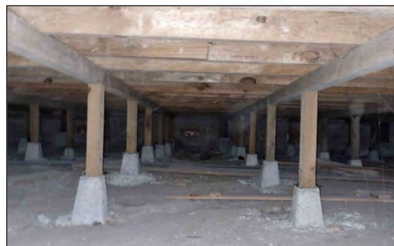
Photo 6: Timber subfloor supporting hall floor
