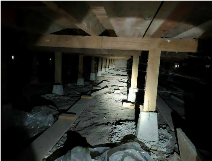
7. Sub-floor beneath the hall
