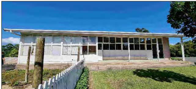
Photo 3: Eastern building elevation
