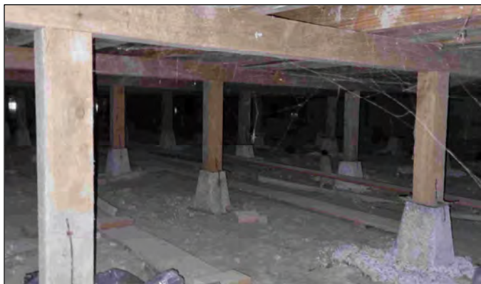
Photo 21: Typical view on subfloor
