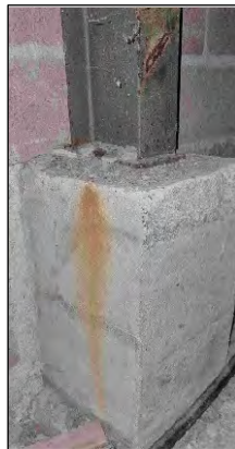
Photo 8: Portal Frame Base
