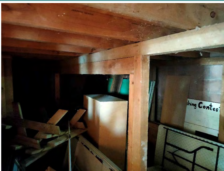
6. Sub-floor beneath the stage
