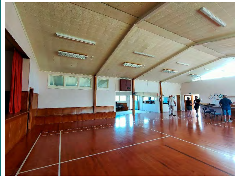
10. The interior view of the hall and steel portal frames (middle span)
