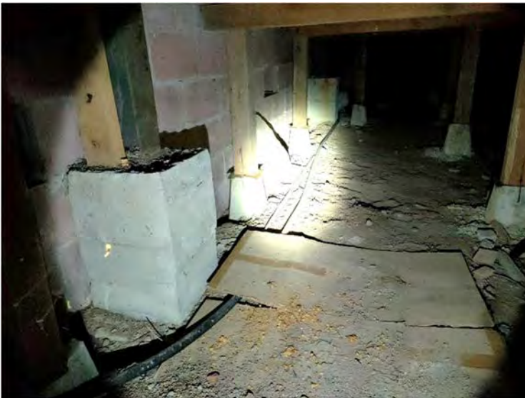
8. The base connection of the UB portal frame in the sub-floor
