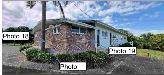
Photo 17: Brick veneer NW elevation
