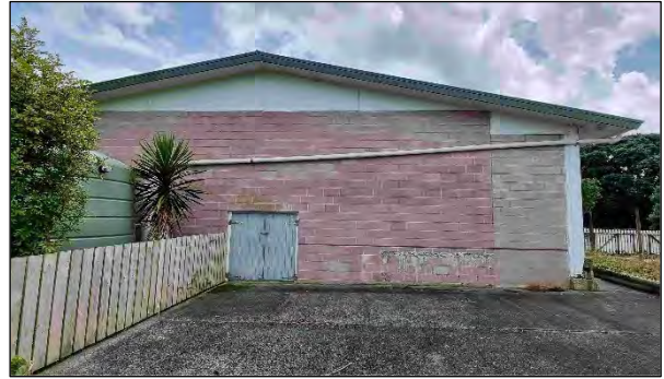
Photo 2: Southern building elevation
