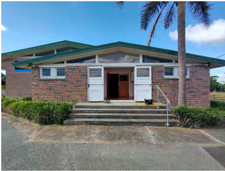
4. Entrant foyer & toilet block (North)
