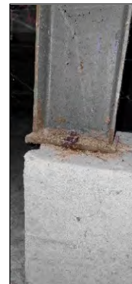
Photo 9: Portal frame base plate
