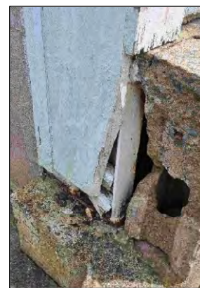
Photo 12: South frame base plate
