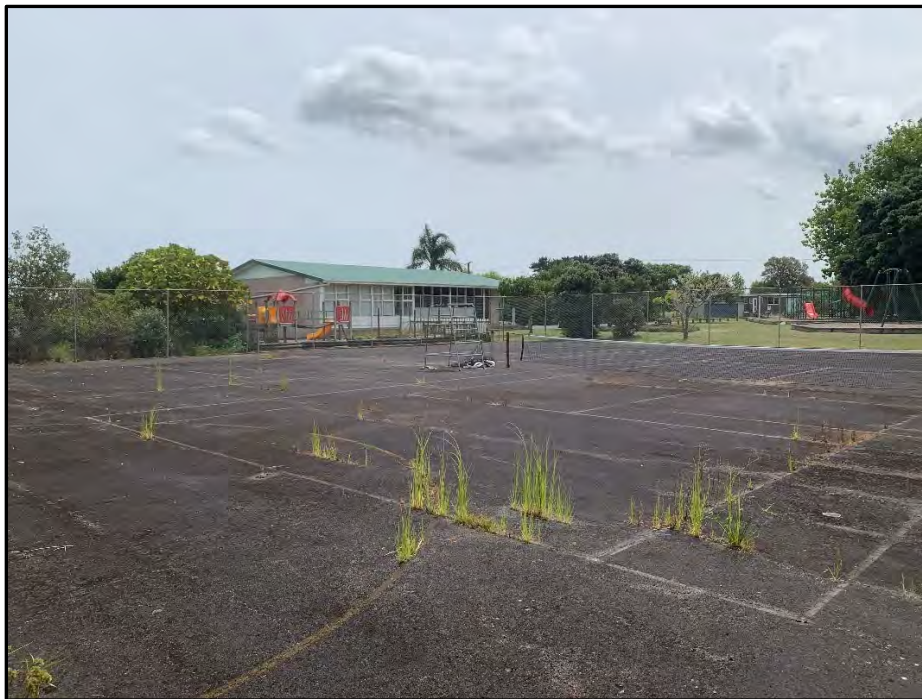
Photo 8 Existing tennis court
