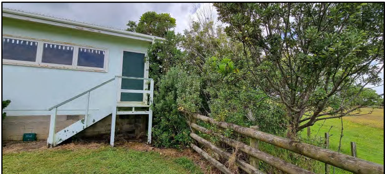
Photo 7 Existing trees within close proximity to hall building
