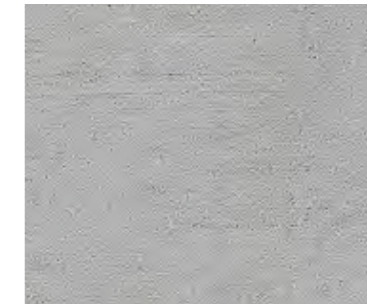
② Standard Footpath Light Broom finish concrete with 4kg/m 3 black oxide (refer civil documentation for buildup details)
