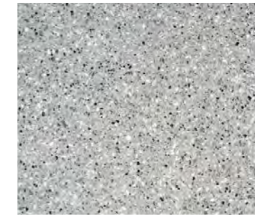
① Shared Path Exposed aggregate concrete with 4kg/m 3 black oxide (refer civil documentation for buildup details)
