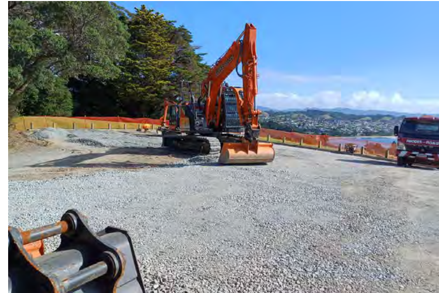
Photo above and below: Base preparation in advance of new concrete pavement
