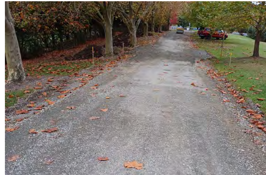
Photo above and below: Base preparation in advance of new concrete pavement
