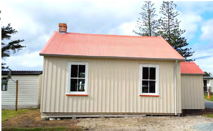
Photos Right: Work nearing completion
