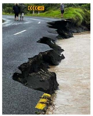
Figure 15: Erosion to Bethells Rd, north of Erangi Rd
