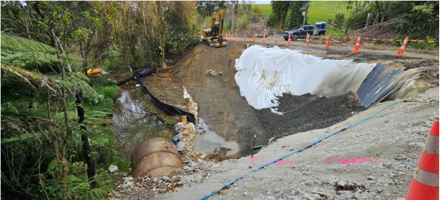
Slip repair underway on Yelash Road
