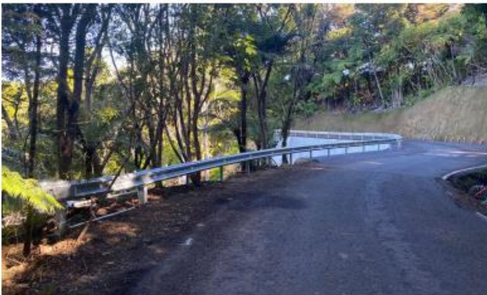
Before and after of one site on Lone Kauri (L5)
