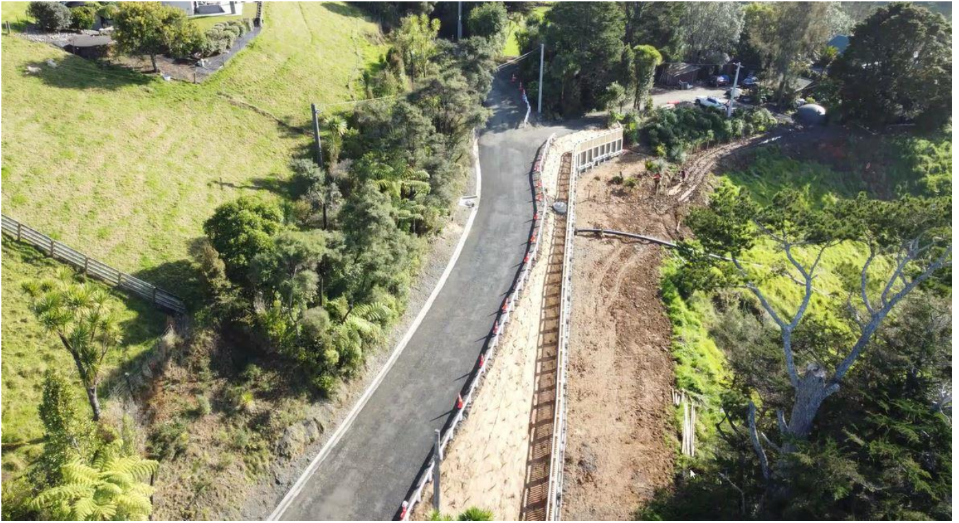
A photo of the finished repair on Caton Road
