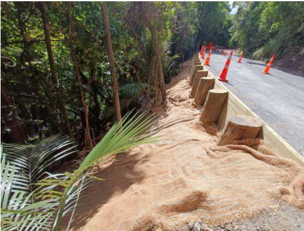
Timber retaining wall on Titirangi Beach Road
