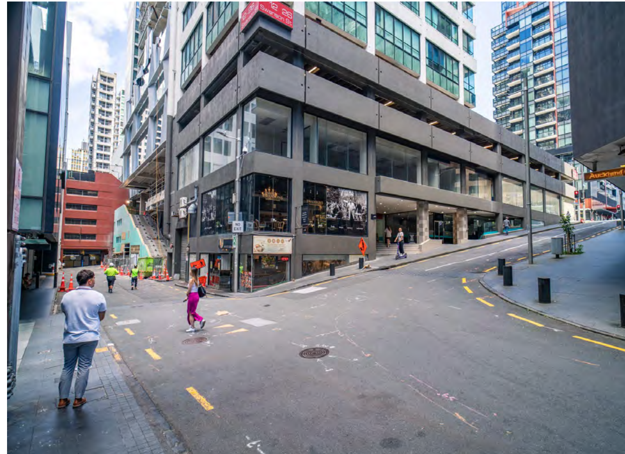
Mills Lane & Swanson Street Improvements
