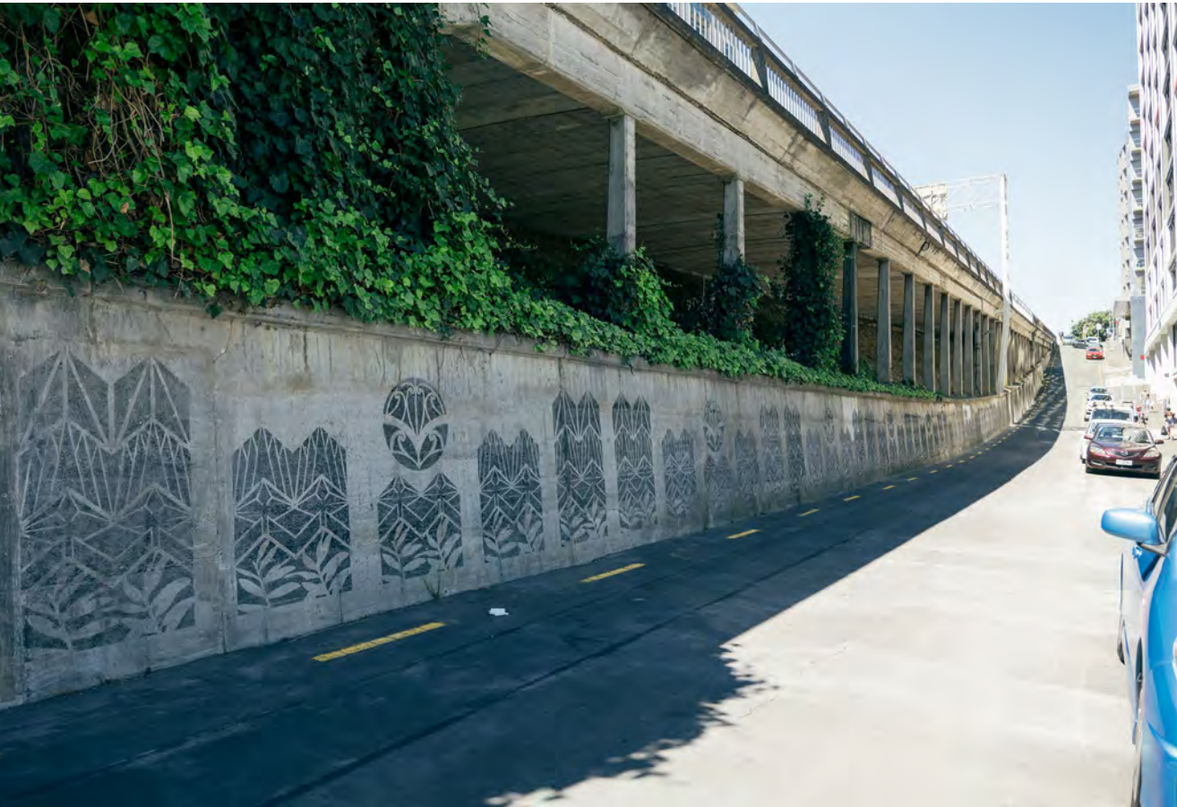
Nelson Street Laneway
