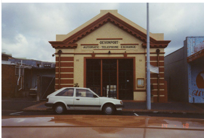
5 Clarence Street, Devonport Automatic Telephone Exchange Building. NSC 891/436.
