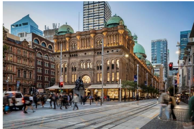
Figure 4 Queen Victoria Building Today
