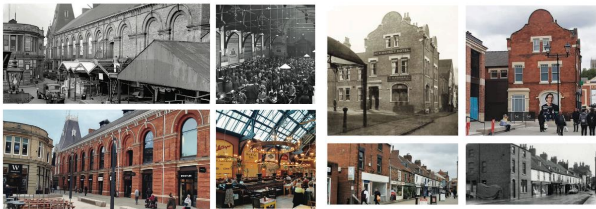
Figure 1 The Cornhill Quarter in Lincoln before and after.
