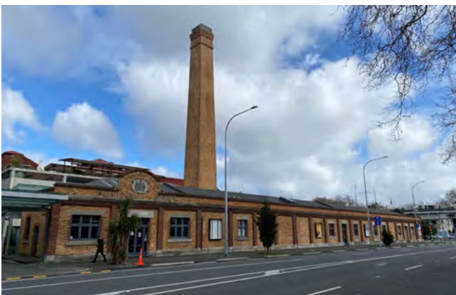
Image: City Destructor Buildings (former), including boiler room, depot perimeter buildings, generator room, battery house, chimney, stables, and destructor building on Victoria Street West, Auckland Central (Category A, ID 02074). It is now used for galleries, workshops, studios, offices, restaurants and retail shops © David Bade (Heritage Unit, Auckland Council, 2024)
