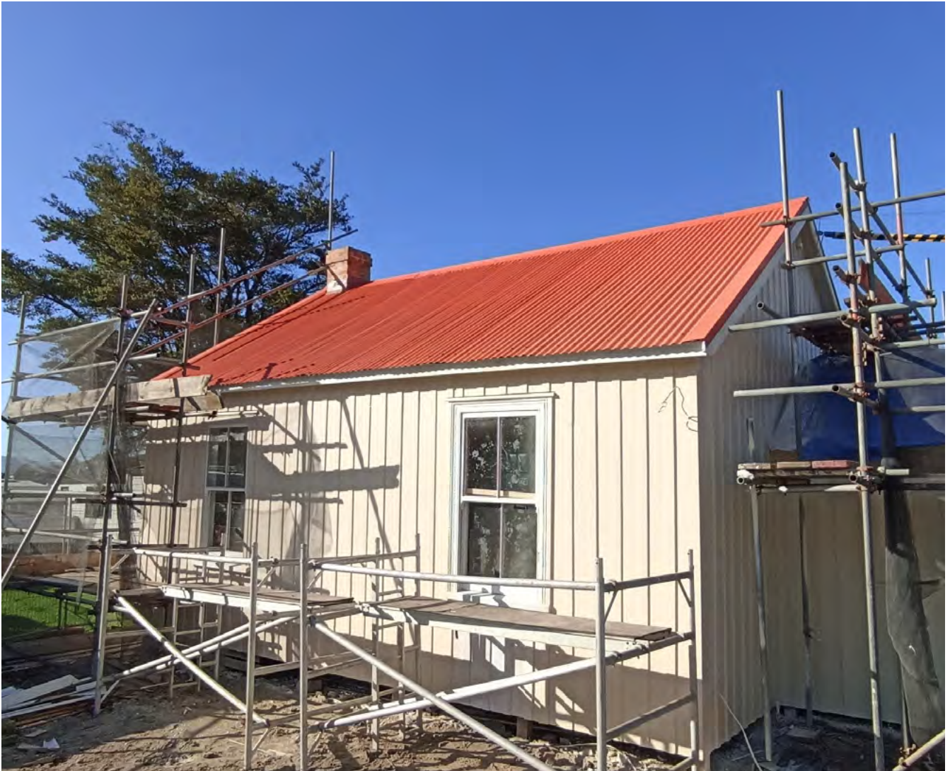
Image: Restoration of the former Sandspit School, Sandspit. Built in the 1880s. © Richard Bland (Heritage Unit, Auckland Council, 2024)
