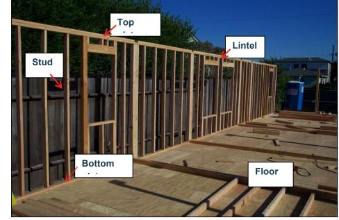
Wall framing comprises studs, top plates, bottom plates and lintels.
