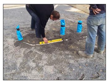
Ideally the certifying drainlayer or a licensed person working under their direction is on site, and an as-built plan must be provided at the time of the inspection.
