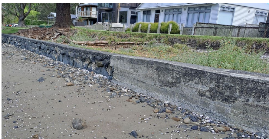
Timber and rock seawalls, Buckleton Beach (Source: Matthew McNeil)
