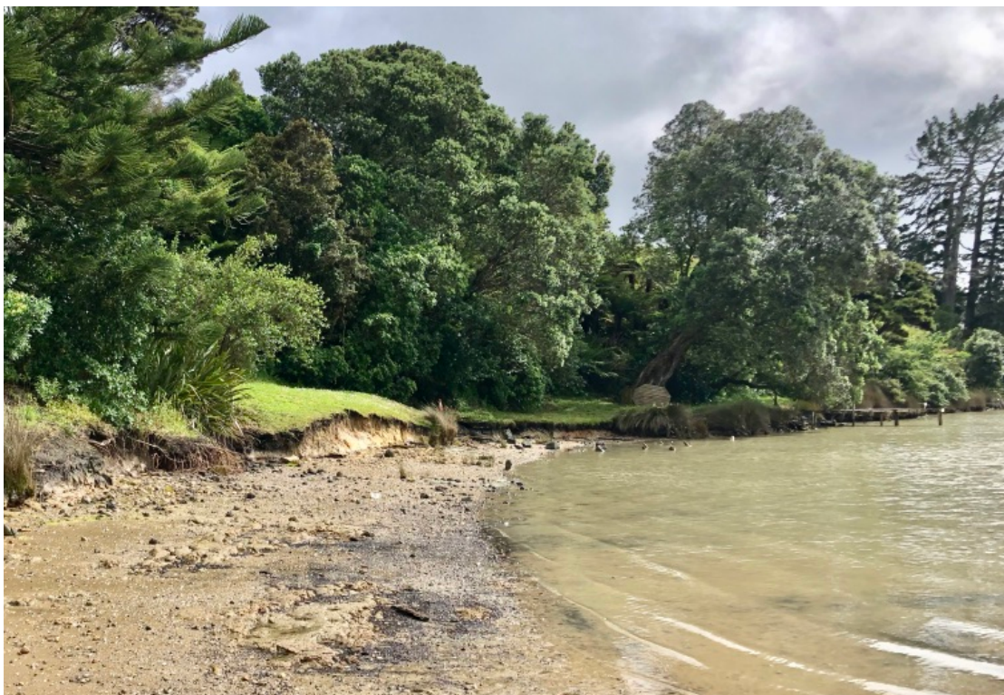
Figure 2 - Kowhai Beach Reserve Nov 2022, 24 years on, no longer a gentle slope to beach, eroded to flax and white post
