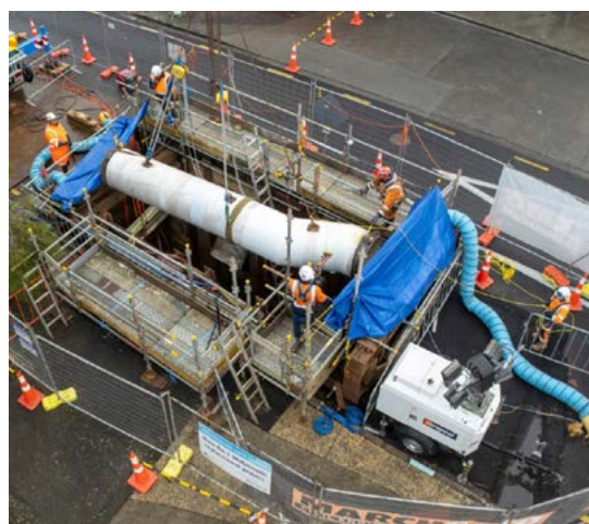
▲ Installation of one of the final pieces of pipeline.
