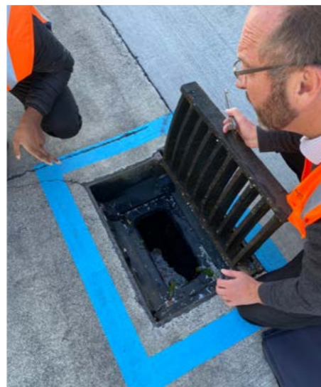
► Pollution prevention team assesses stormwater drain
