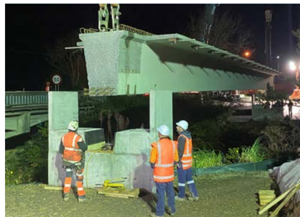
▲ Lifting the footbridge into place at Rodney Street, Wellsford
