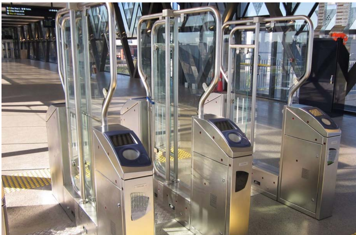
New electronic ticketing gates at Ōtāhuhu station
