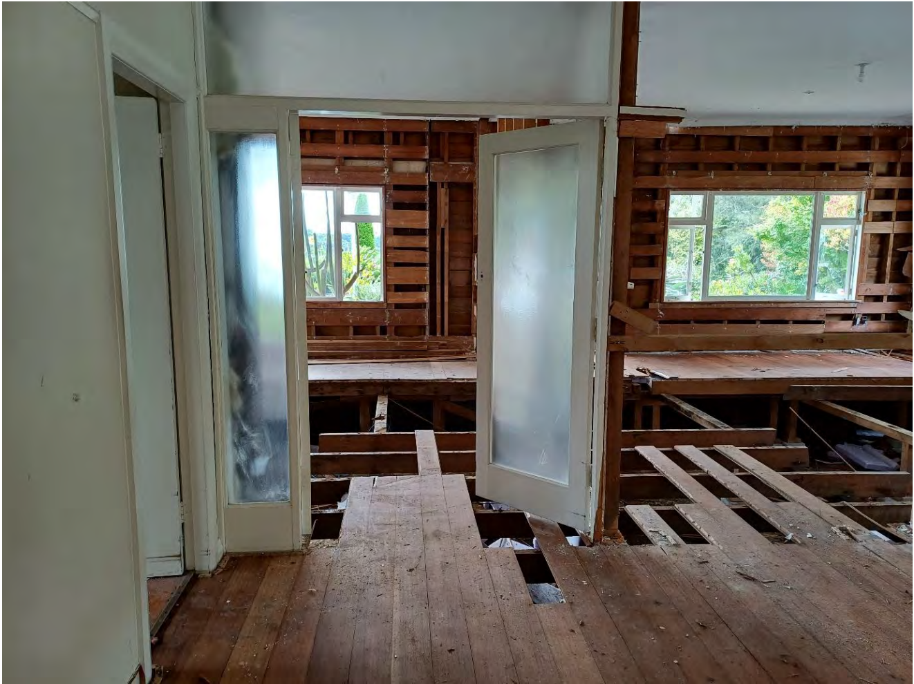
Photo of a house deconstruction project
