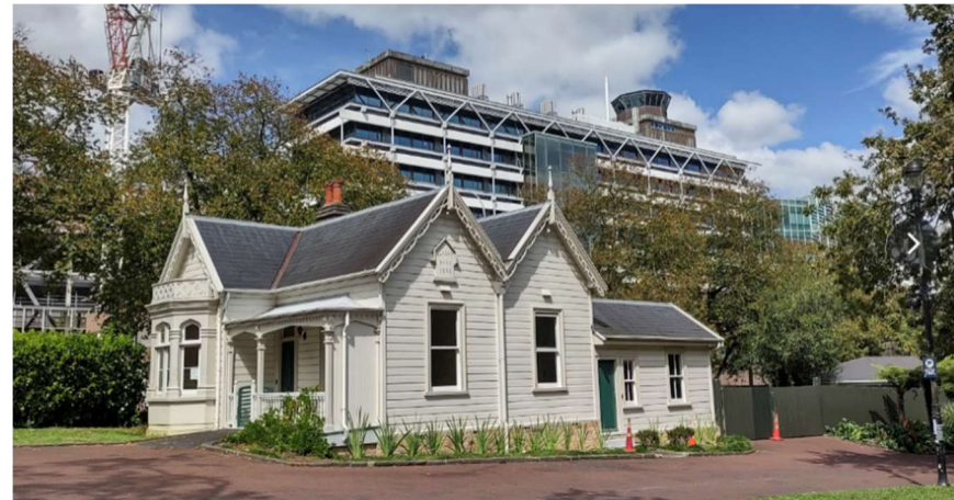
Figure 14 Caretakers Cottage used as a community hub for The Kitchen Project
