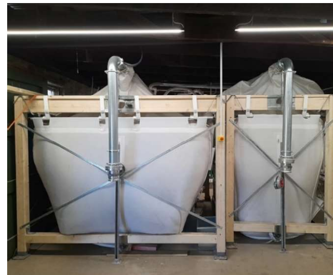
Figure 7 12 tonne capacity pellet hoppers with sloping floors
