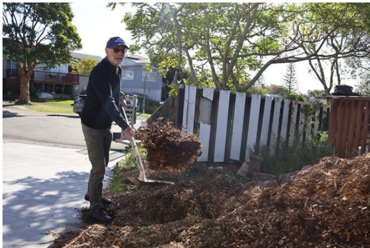
Figure 10 Mayor Wayne Brown shovelling bark from a blocked manhole
