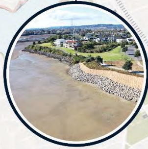
Drone shot of revetment
