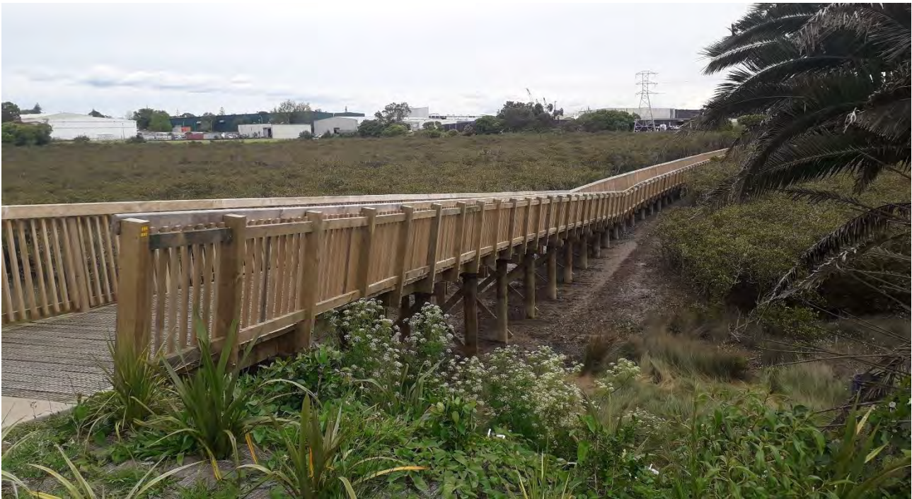
Figure 5-15: Norana Boardwalk, Māngere inlet. Photo credit J Morriss
