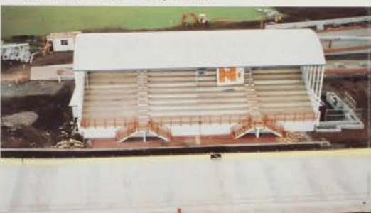
Grandstand at Completion
