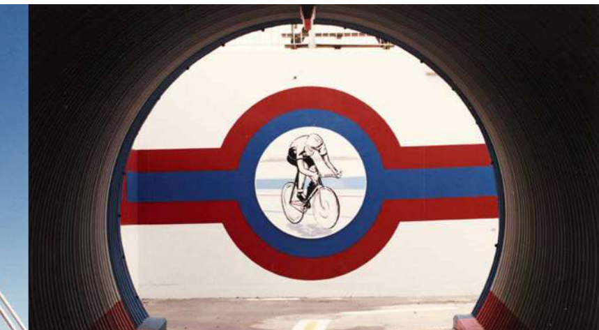
Entrance to the cyclists subway at the velodrome. Photograph taken during the later stages of construction, 1989
