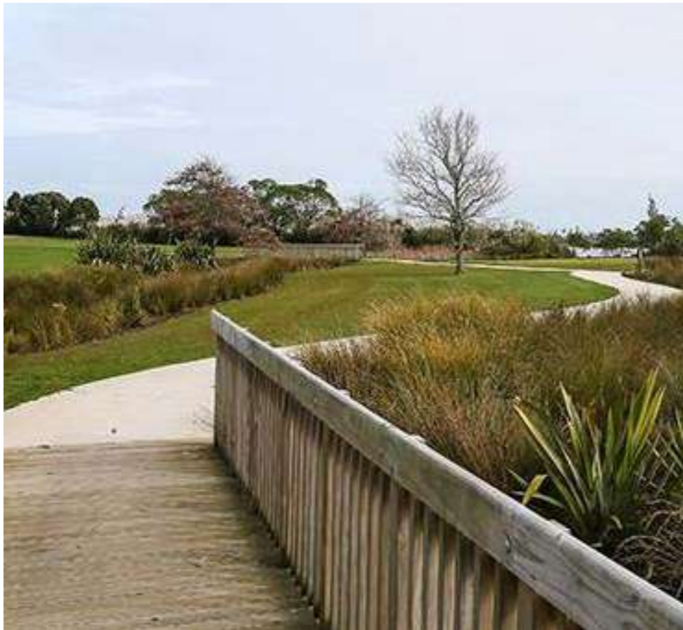
Timber bridge crossings through riparian planting
