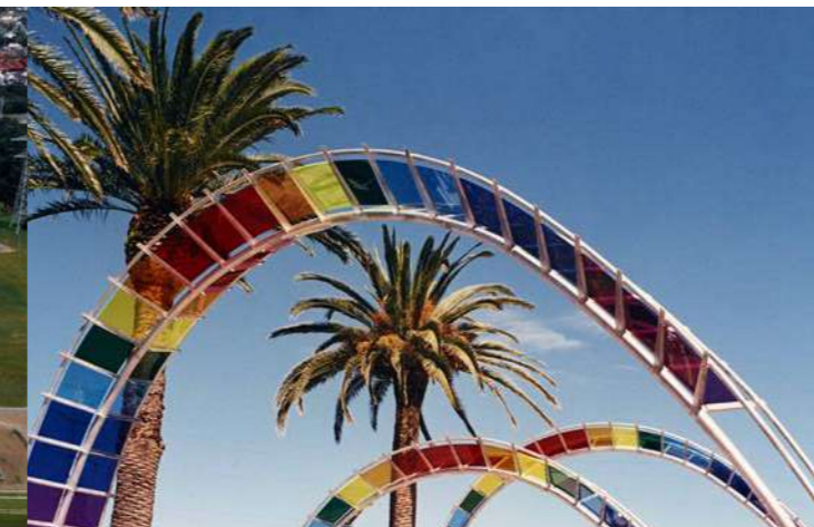
Entrance feature at the velodrome at Manukau Sports Bowl constructed from tubular steel and coloured Perspex panels, 1989
