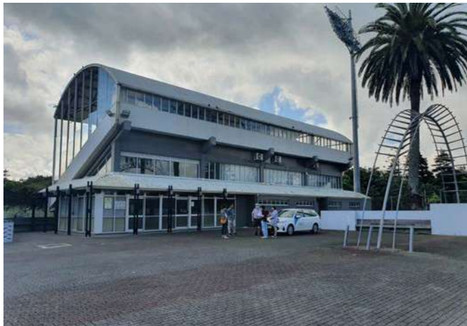
The velodrome grandstand from the concourse
