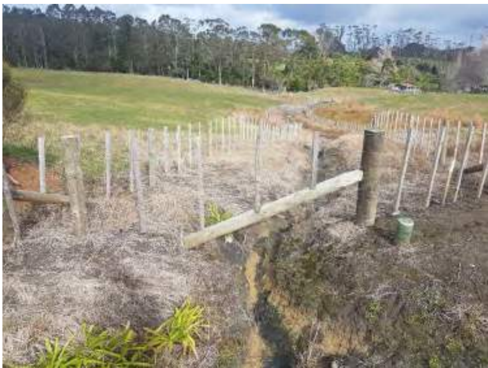
Photo 1 – Flow Path looking South from edge of Sandspit Road
