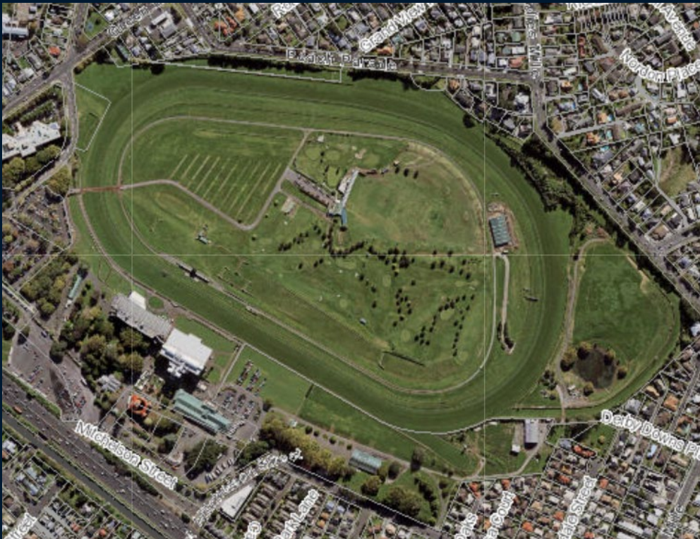
Aerial View – Ellerslie Racecourse
