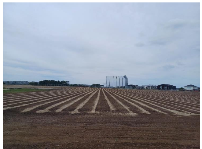
Photo: Sand slit drains installed for fields 2 and 3, December 2024
