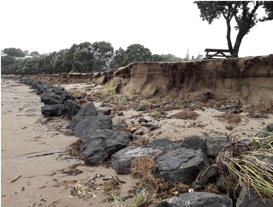
Fig 7: Storm damage at the eastern end of Stanmore Bay, Jan 2018
