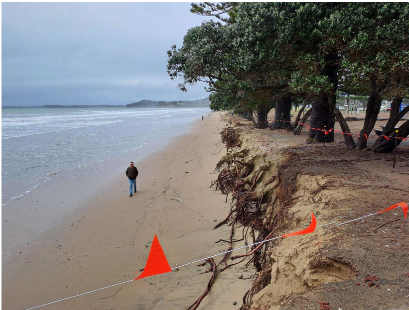
Fig 2: Storm damage at the northern end of the reserve following Cyclone Gabrielle, Feb 2023
