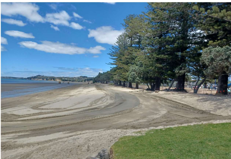
Fig 3: The northern end of the reserve after sand transfer work
