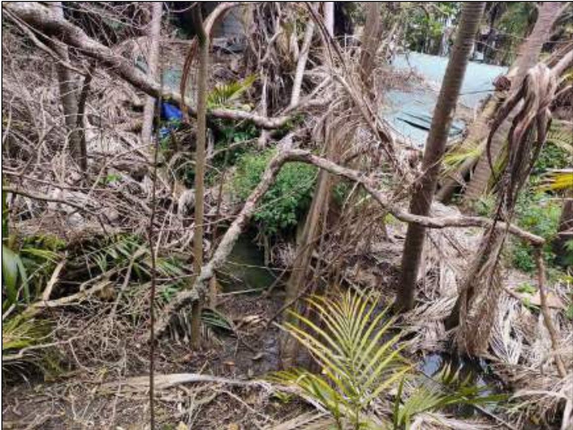
Figure 2.9 Ponding of water on top of the landslide debris at the rear of the dwelling, looking west.
