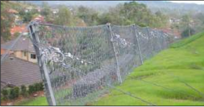
Figure 4.1 Example of proprietary flexible debris flow barrier
