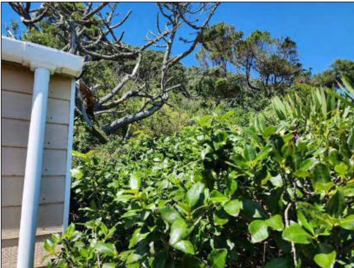
Figure 2.2 Steep vegetated slope at the rear of the dwelling
