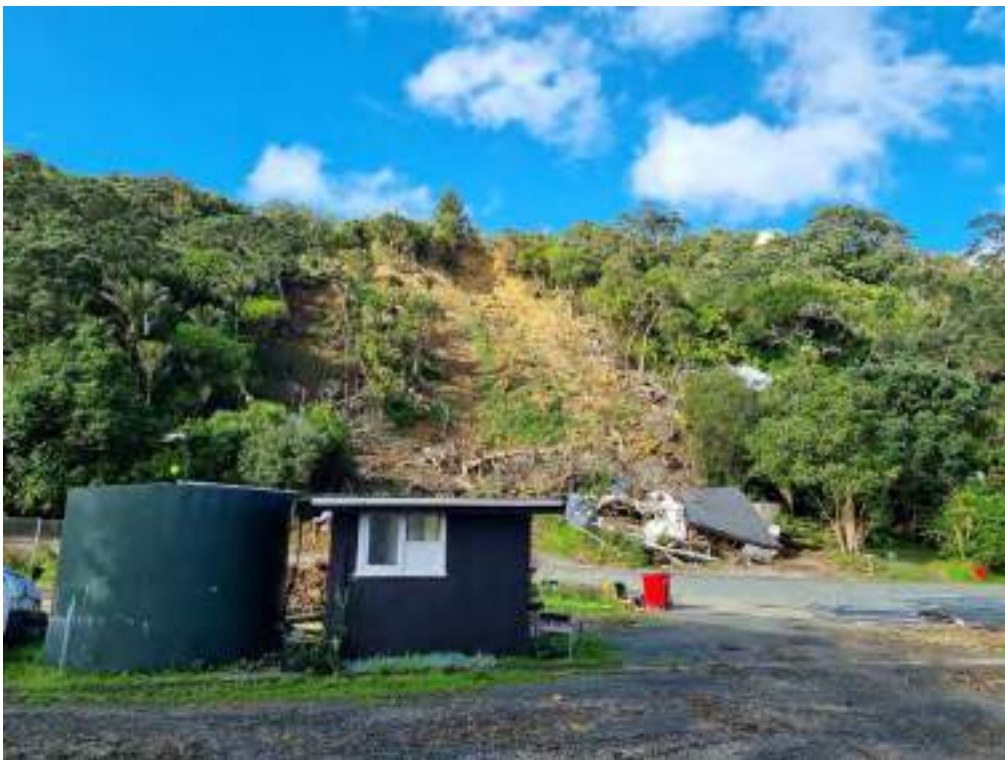
Figure E3 View of same dwelling pictured in Figure E2 showing overall view of landslide with accumulated vegetation at toe of slide.
