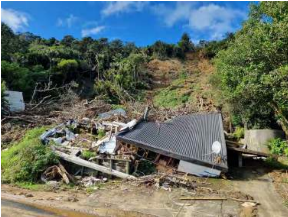
Figure E2 Example of a dwelling completely destroyed on Motutara Road where two fatalities occurred.
