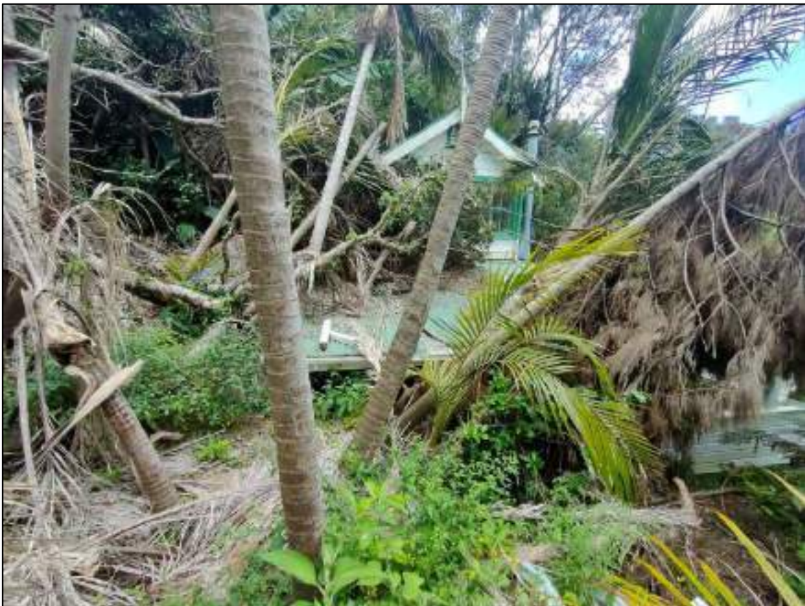
Figure 2.8 Close to the lateral extent of the landslide debris at the rear of the dwelling, looking southwest.
