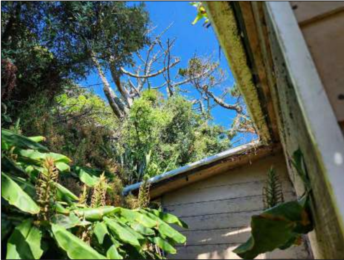
Figure 2.1 Steep vegetated slope at the rear of the dwelling
