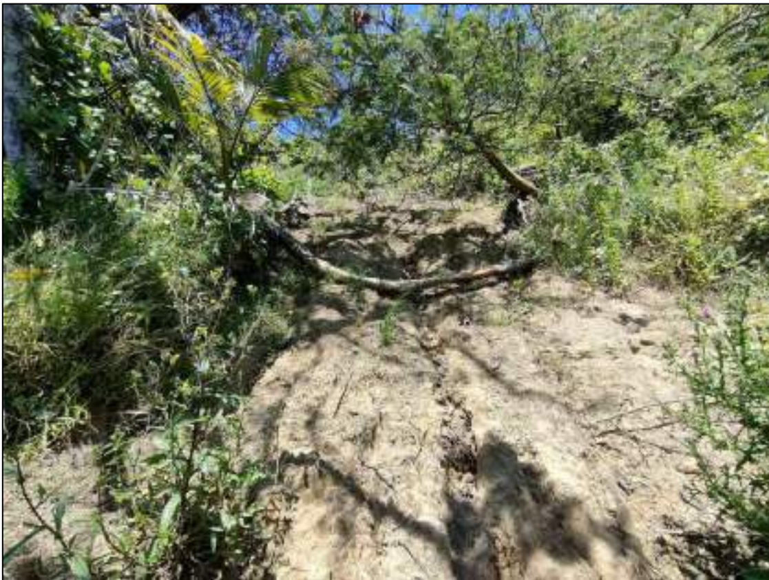
Figure 2.9 Failure surface (evacuated zone) exhibiting evidence of post failure erosion. Looking upslope.
