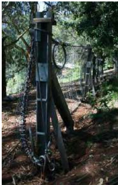
Figure 4.2 Example of a pressure post that can be used at the end of flexible barriers that may be used at property boundaries
