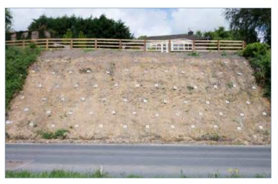
Figure C-6 Example of surface erosion prevention matting and mesh for use with soil nails on relatively steep slopes.
