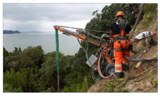
Figure C-5 Example of typical small, roped access rig used to install anchors or nails on steep slopes.
