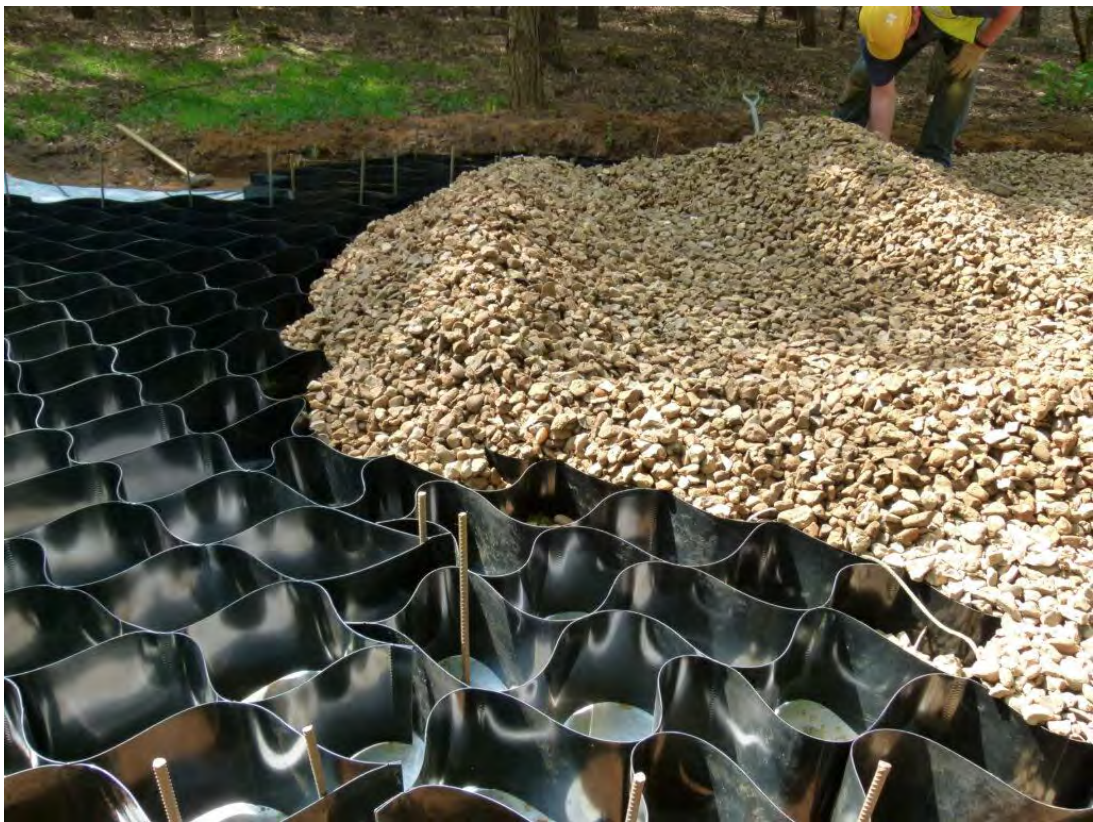
Figure 3: An example of a cellular confinement mesh (ABG Geosynthetics)
