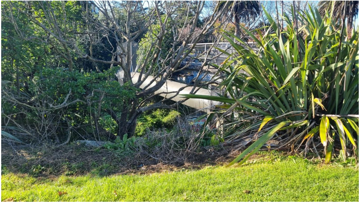
Figure 17. View looking east along the existing Walmsley Road bridge crossing
