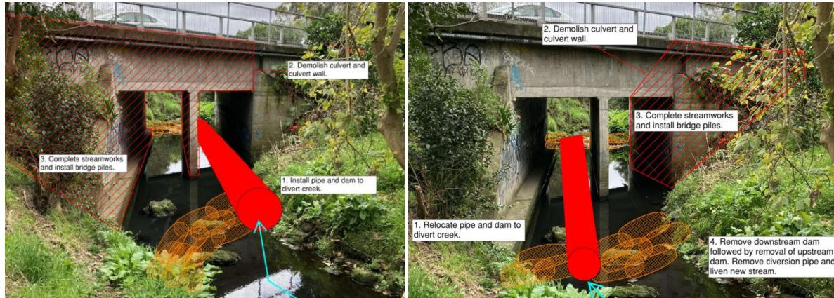
Figure 3.2: Two stage stream diversion and culvert demolition.
