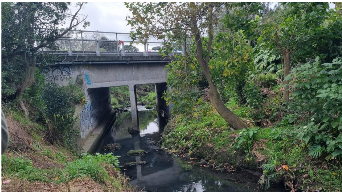
Figure 2.2: Te Ararata Creek Culverts.
