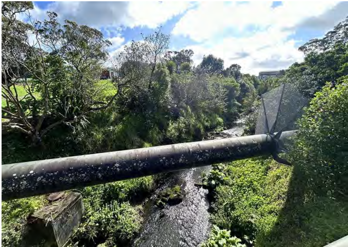
Photograph Appendix B.4: View facing north of water pipeline.
