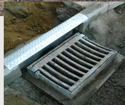
New back-entry catch pit
